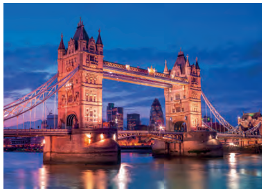
Cod. 39674.0 Tower Bridge
